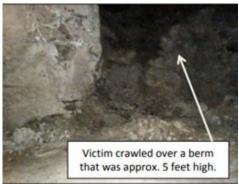
On January 25, 2017, a miner was found in an underground limestone mine after failing to exit the mine at the end of his shift. The miner was found under material that had fallen on him from a rib in an area of the mine that had been barricaded to prevent entry due to bad roof and rib conditions.
